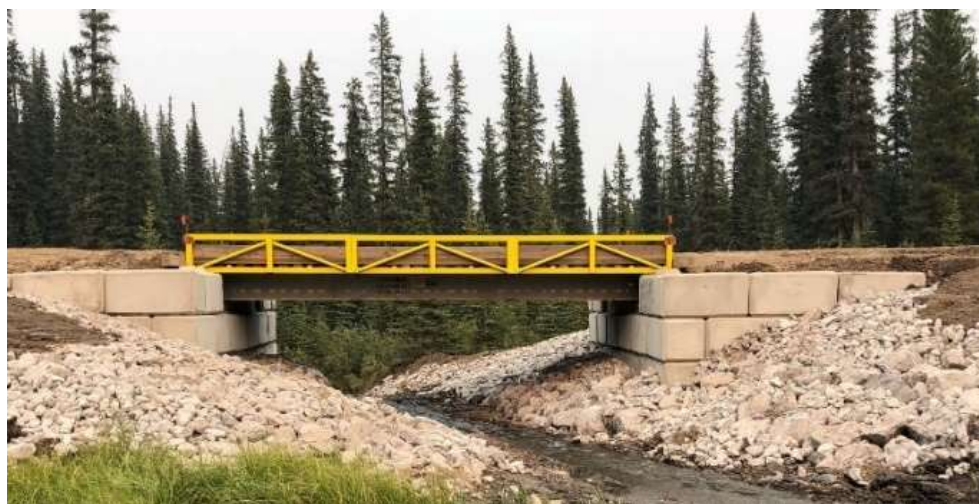
Example of watercourse crossing management in the Edson area
