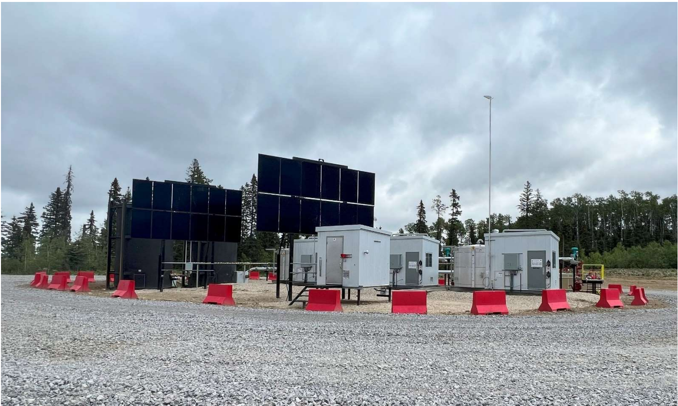
Typical Peyto multi-well pad measurement buildings equipped with solar panels, integrated water tanks, remote monitoring, and emergency shutdown equipment designed to minimize footprint while providing safe, reliable operations.
