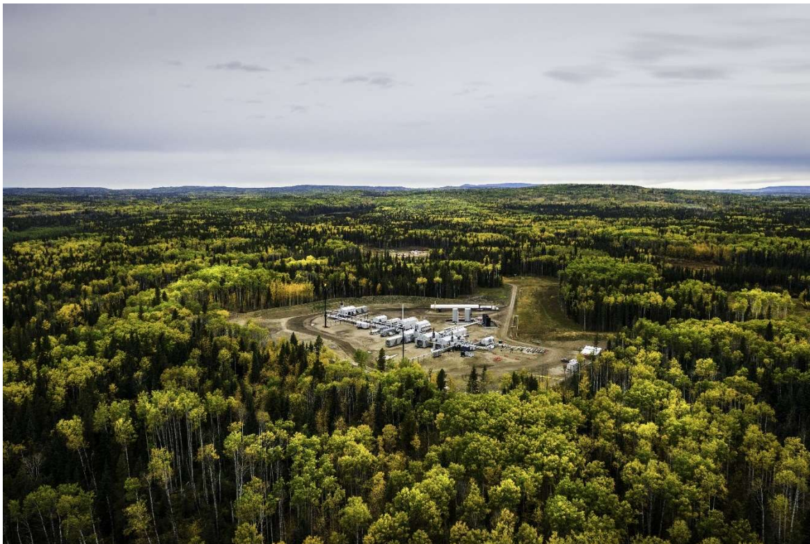
Peyto Swanson Gas Plant, Edson AB
